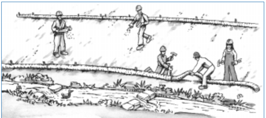
Drainage swales channel runoff around a construction site. Planting temporary vegetation on freshly graded areas, and trenching and staking fiber rolls and/or silt fences downslope are common techniques for preventing erosion and controlling sediment.
